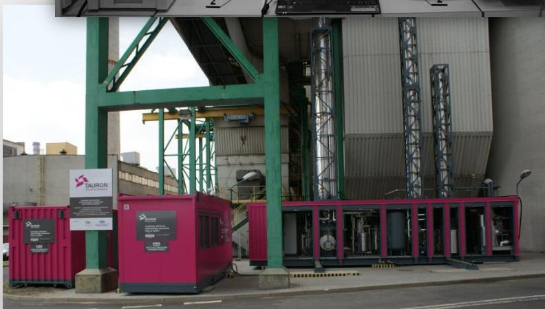
PDU for CO<sub>2</sub> capture process – 100 m<sup>3</sup>/h
