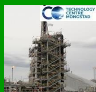
TCM Mongstad Norway 40 MWth, Chilled Ammonia, CHP & Refinery Offgas (RCC)
