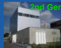
COORETEC DE, FP7 EU - Darmstadt Germany - 1 MWth Regenerative Calcium Cycle - Coal
